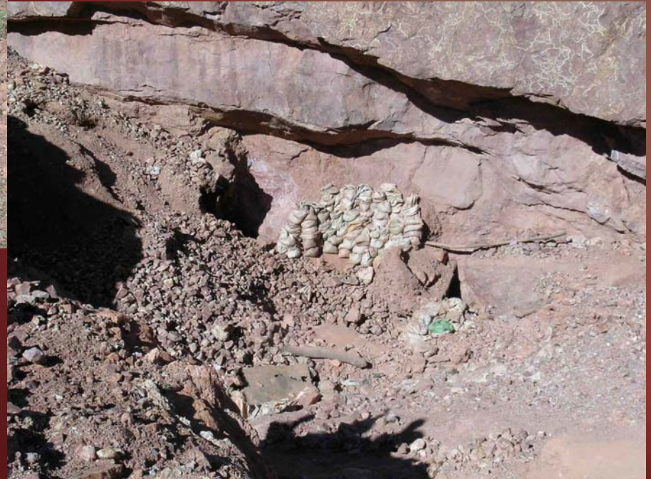
Recent rock collapse on left & rock overhang
